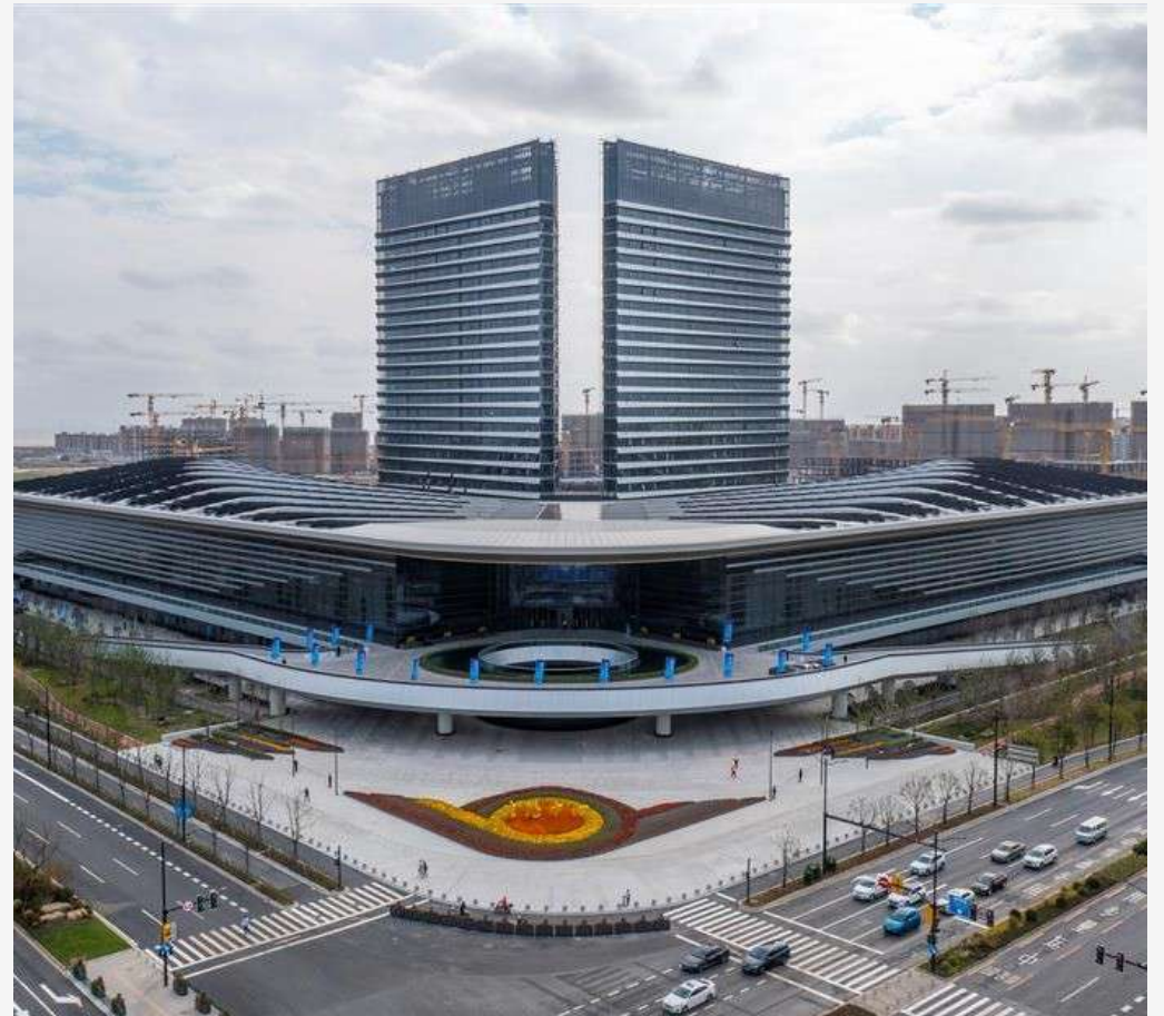
The World Laureates Forum, Shanghai — ~900 t Custom Steel, 28 m arc spans
